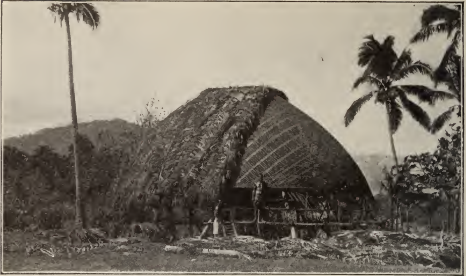
BUILDING A SAMOAN HOUSE
